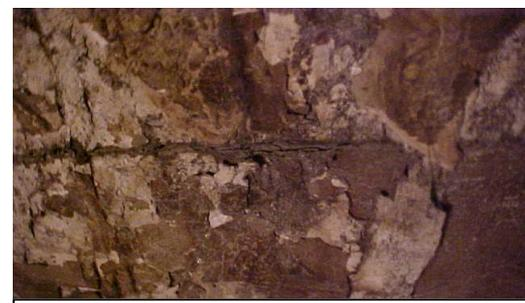
Figure (8) loss of some architectural elements as a result of biological attack at the ceiling **a** bat droppings **b** extracts of birds **c** Bees nests
