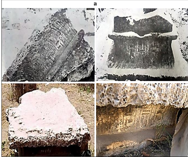
Figure (5) a. the shape of the stone cornice at the time of detection and it appears in an up side down position, b. the shape of the stone cornice, 2022. Tafoni or honeycomb aspects are shown at the top of the stone cornice.
