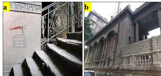
Figure (1) Shows a. graffiti on the staircase, b. added bricks
